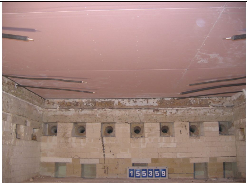
The exposed face of the ceiling assembly prior to testing
